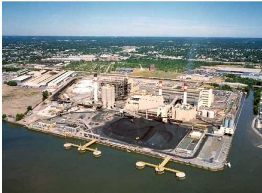
Figure 1 Eddystone Generating Station (Source: Eddystone Application and Conservation Plan)
