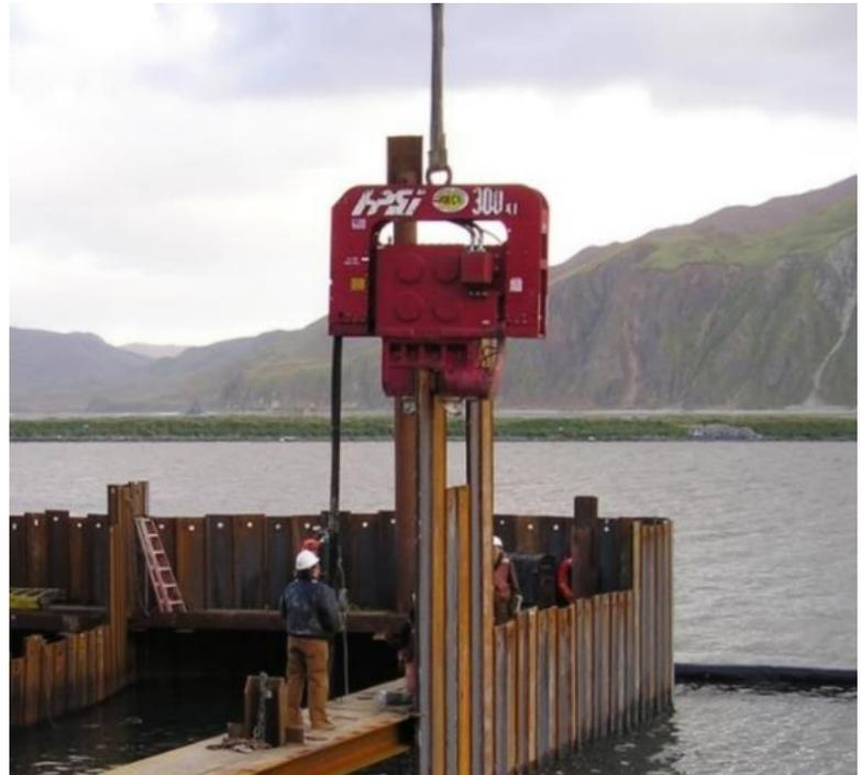
Figure 3. Installing sheet piles with a vibratory hammer.
